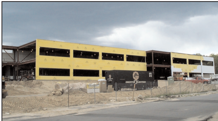
New Facility - Front elevation (May 15, 2001)
